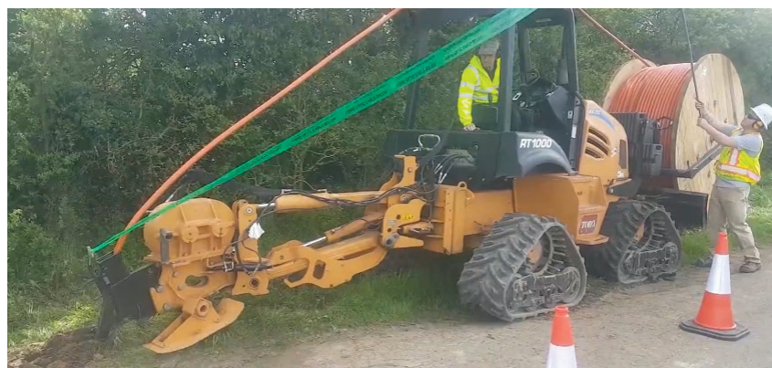
Emtelle's fibre and duct solutions have been used by Gigaclear since 2017 for providing spine, distribution and drop connections to residential and commercial premises, mainly in rural districts
